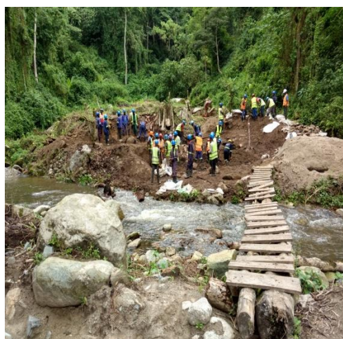
Excavation at the project site
