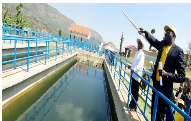
Commissioning Lirima water treatment Plant and Ground breaking for Lirima Phase II in Namisindwa District: Commissioner, Rural Water Supply Department, explaining the design to H.E. President Yoweri K. Museveni
