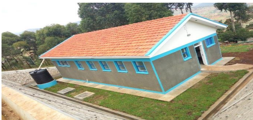
Gender Segregated Water Borne Toilet with 10 stances of which two stances are for disabled and bathroom for girls constructed at Tulel Secondary School in Bukwo District
